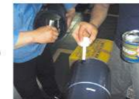
Quickly inserting the fitting after the second application of adhesive
